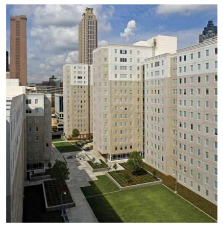
Three finishes were used on the precast concrete panels, comprising a white sandblast finish across the top of the majority of the buildings; a buff sandblasted finish below that on the bulk of the buildings; and inset thin bricks, used at pedestrian level.
